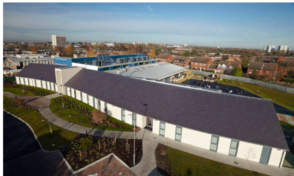
St. Anne's Catholic Primary School, Solihull (with TSH Architects)
