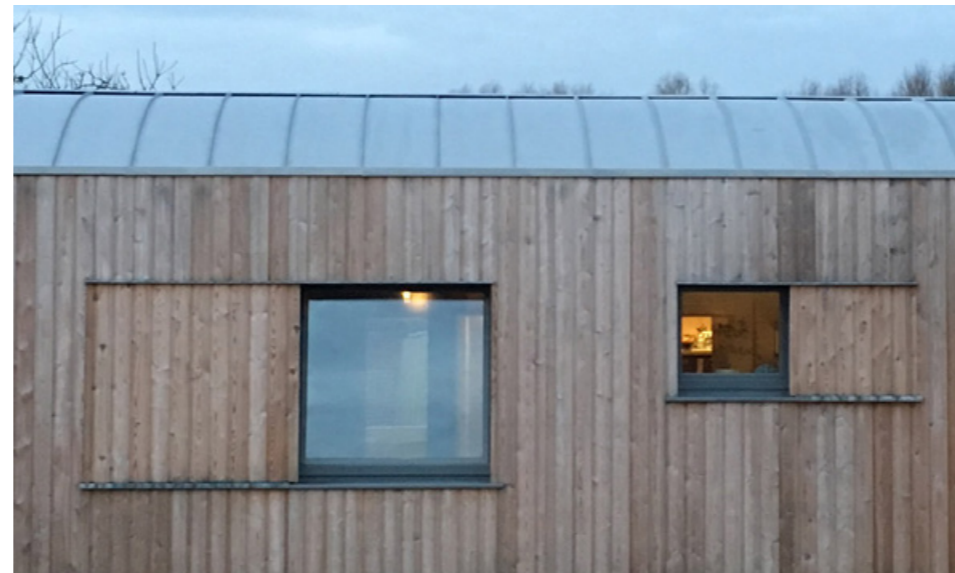
Sliding shutters over south facing windows to control solar gain. Highly insulated on-site timber frame construction
