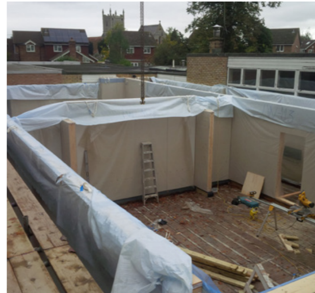
Off-site fabrication used on a primary school extension to minimise time on site
