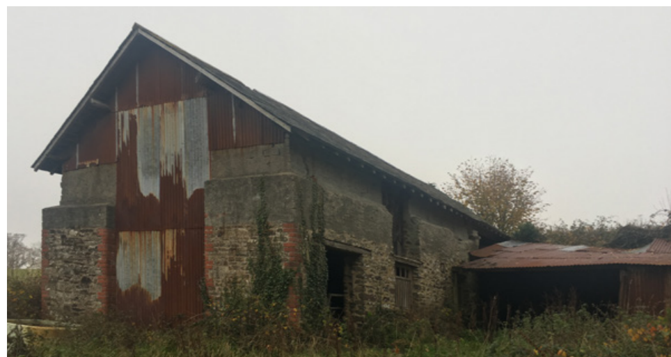
Exterior photo - before
