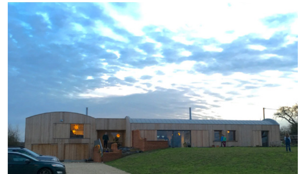
New dwelling to the passivhaus standard, Oxfordshire (with TSH Architects)
