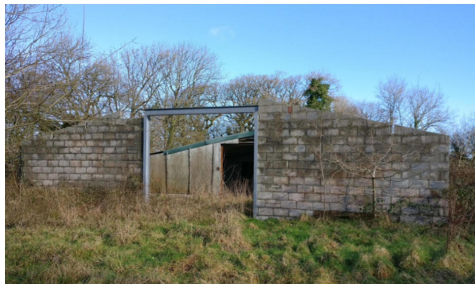
Exterior photo - before
