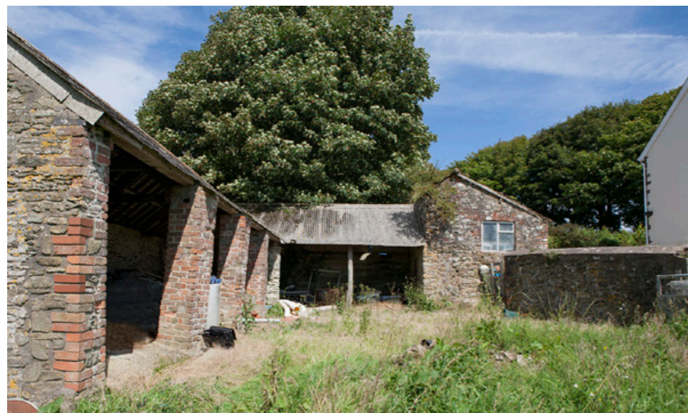
Exterior photo - before
