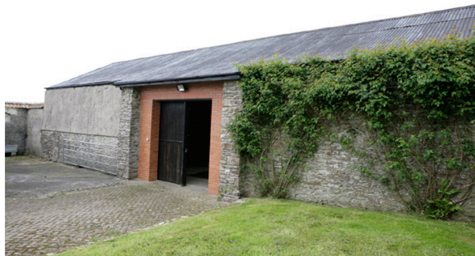
Exterior photo - before
