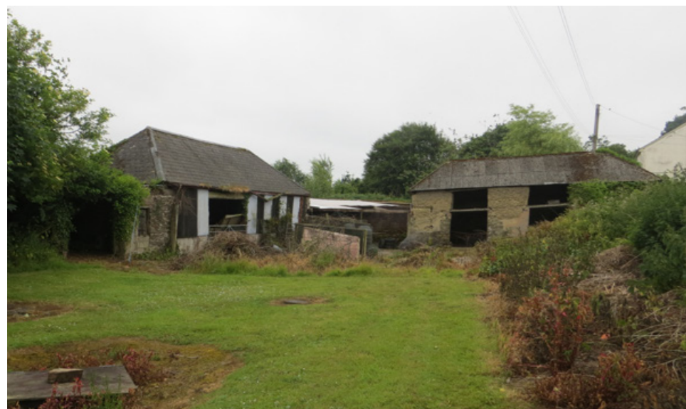
Exterior photo - before
