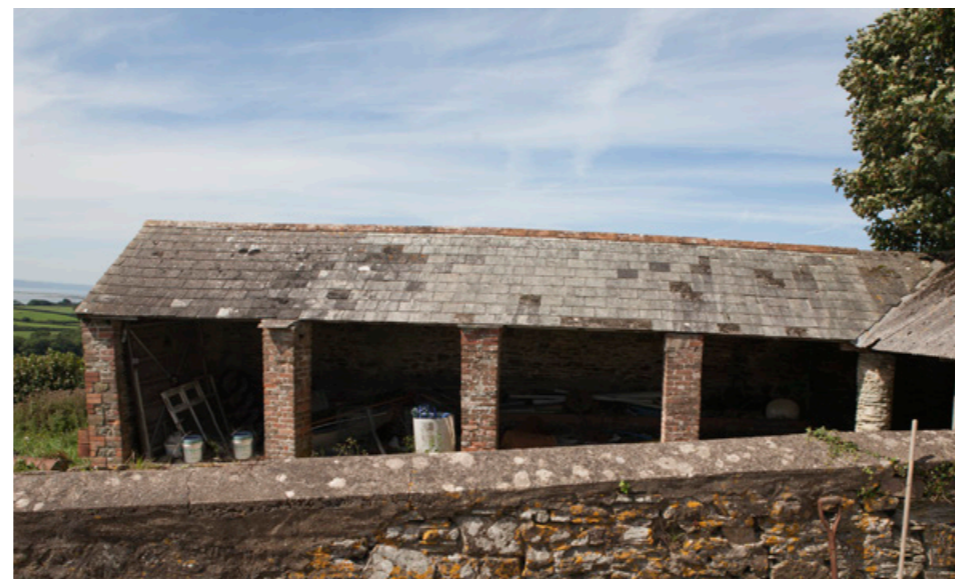
Exterior photo - before
