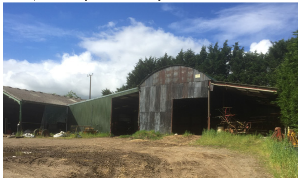
Exterior photo - before
