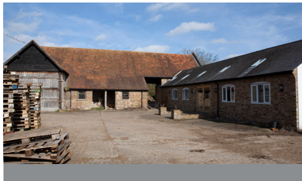
Exterior photo - before
