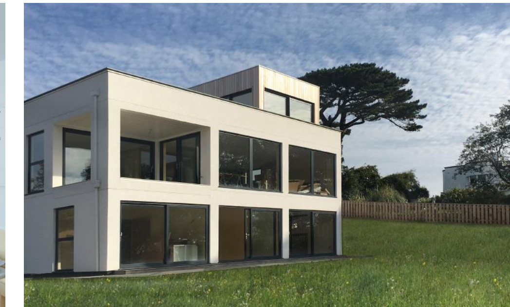
Building almost completed
