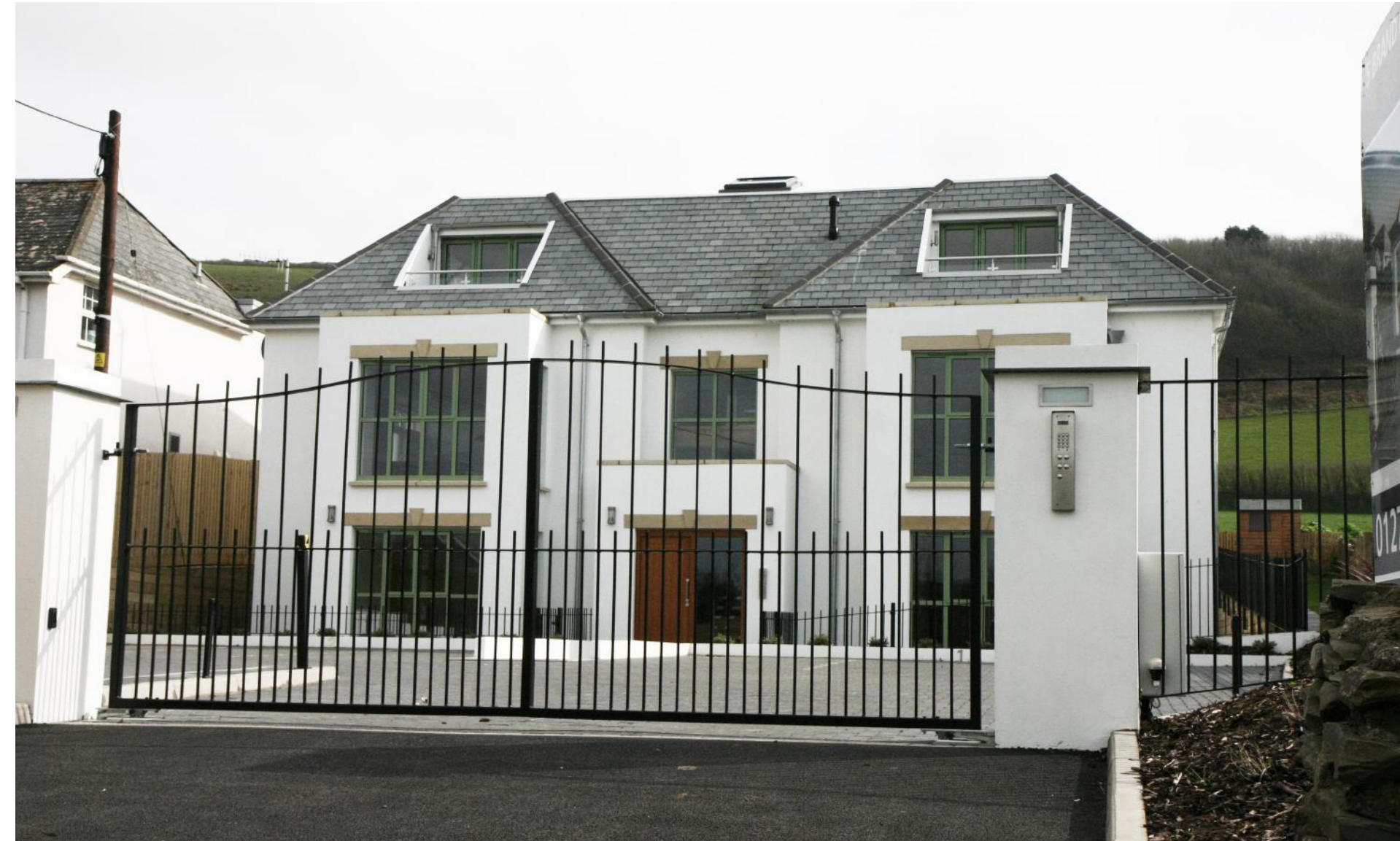
Photograph of completed building
