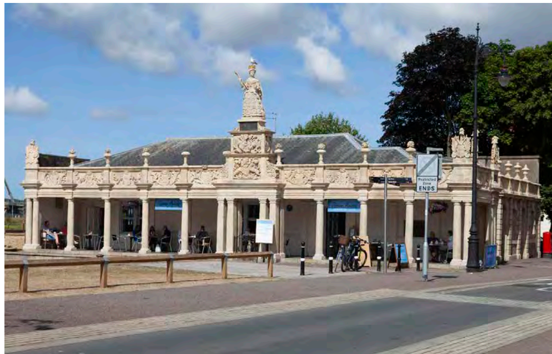
The colonnaded elevation fronting the square has been carefully cleaned
