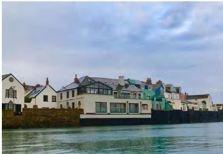
Refurbishment of Grade II listed riverside restaurant
