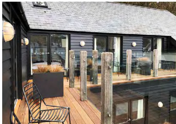
A new terrace was formed for first floor bedrooms
