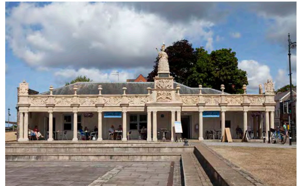
Grade I listed quayside, carefully restored and converted to new restaurant
