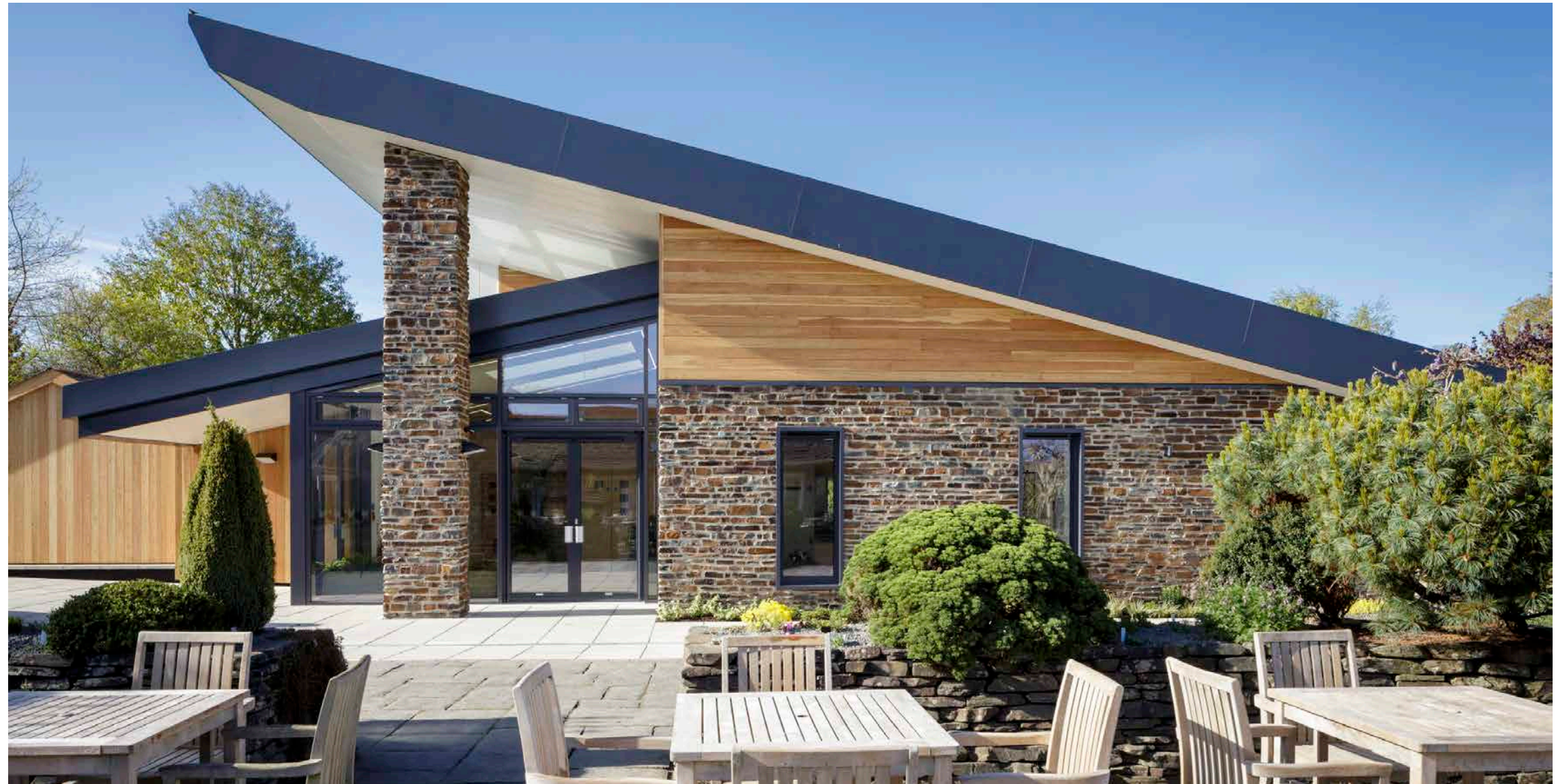
The new Garden Room viewed from the existing restaurant
