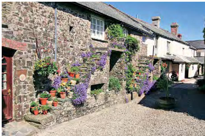
Existing cottages being internally refurbished and conserved externally
