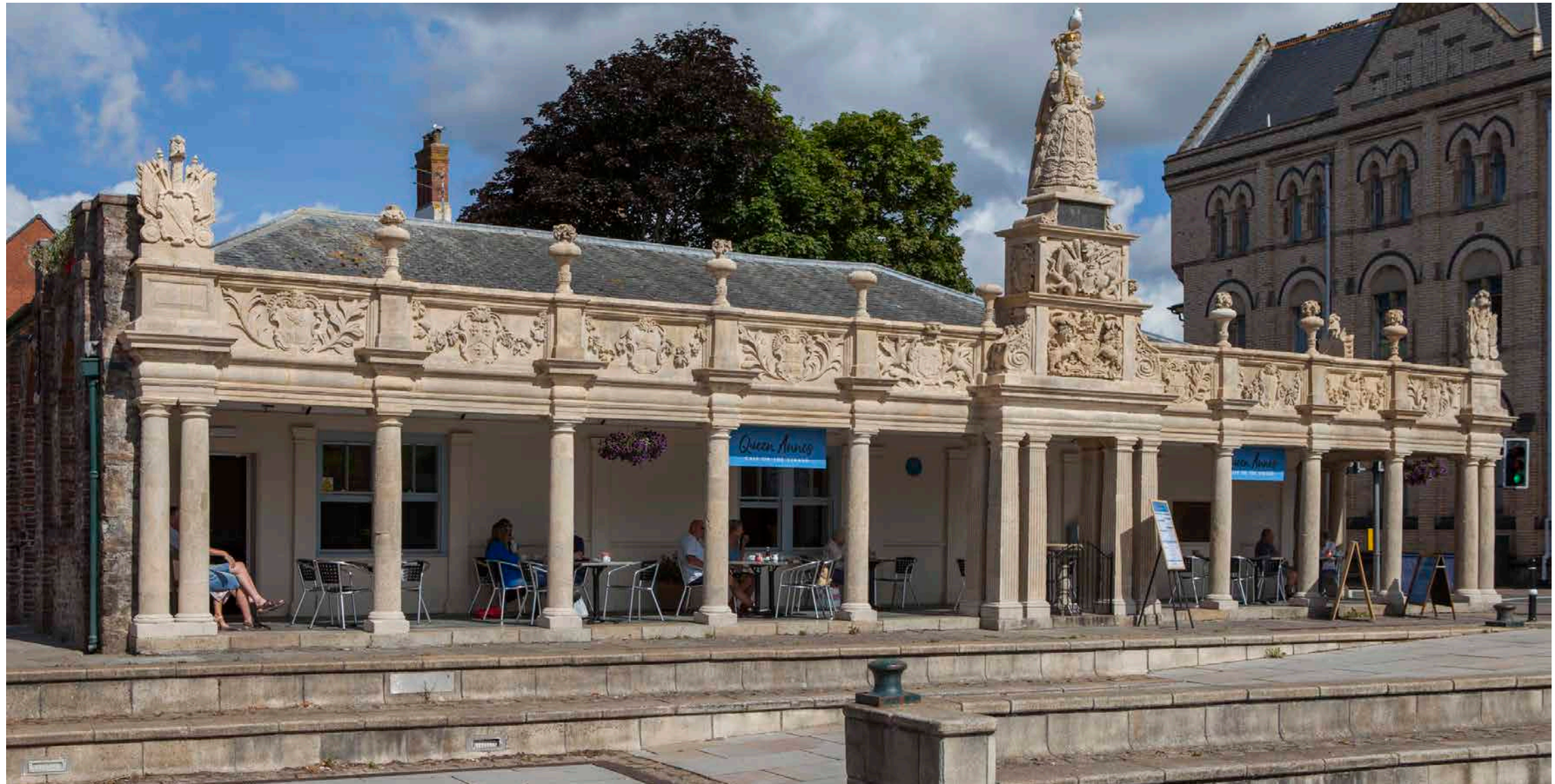
This listed building had been empty for a number of years. The careful conversion and restoration has given the building a new lease of life
