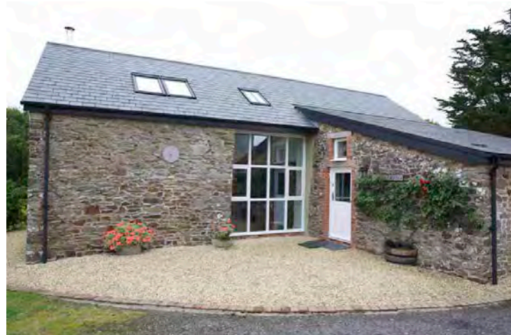
Barn conversion creating a new home
