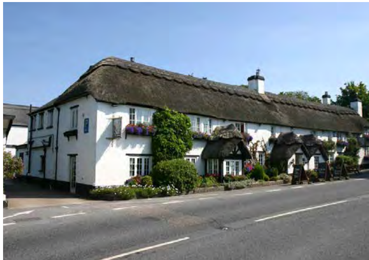
Refurbishment of Grade II listed public house
